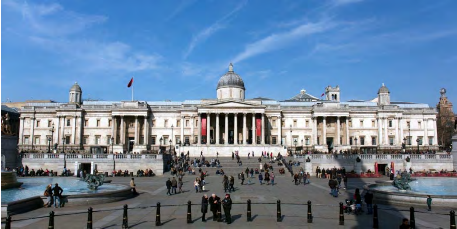
1824– National Gallery in London (The new wing was added in 1869)
